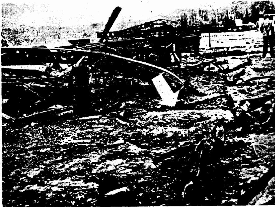
ALPHA SECTION seen from direction of the Assembly building. Explosion apparently originated between launching position four at far left and launching position three at center. Arrow points to crater about three feet deep where nose and center warheads removed from missile that was being modified are believed to have been placed. Metal framework has all been extensively perforated by pellets from exploding warheads. (Aviation Week Photo, June 2, 1958) Figure 46
