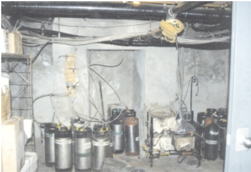
Basement fireplace support south wall near southwest corner (Doug Crompton 12/6/97)
