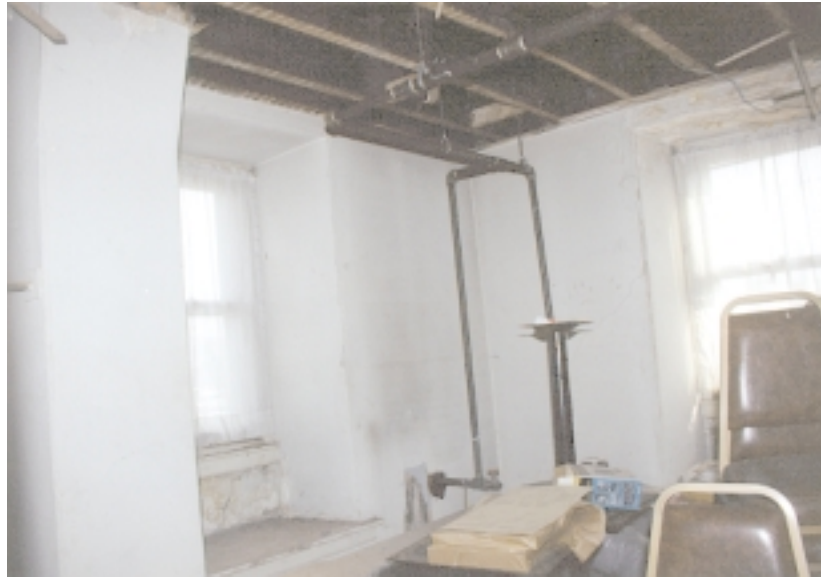
Northeast corner room attic, dormer windows (KAA:97-15/9) 12/6/97
