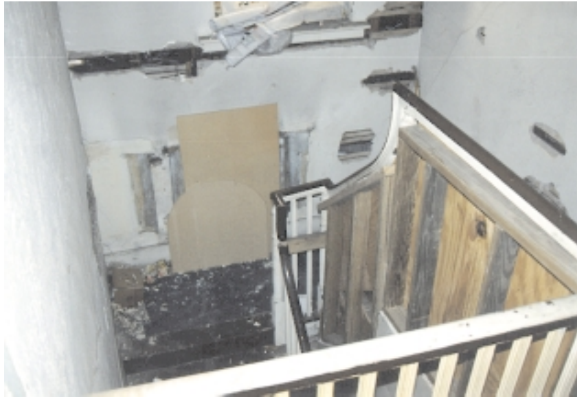
Stairwell to attic, portions of original balusters and railing. (Doug Crompton 12/6/97)
