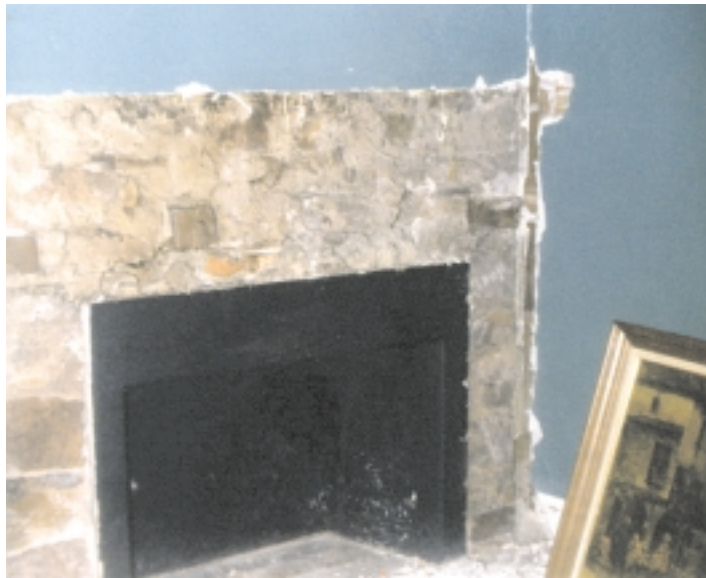
First floor, Southwest corner fireplace (Constance Gerhart 12/6/97)
