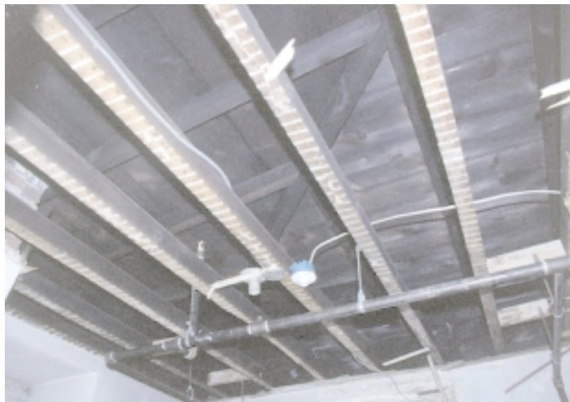
Northeast corner room attic, view of roof construction (KAA:97-15/8) 12/6/97
