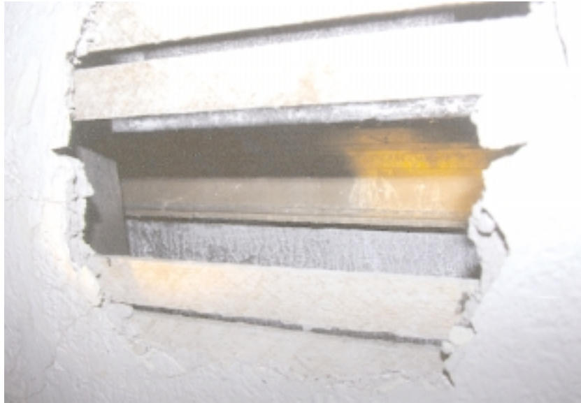
West, stairwell wall to attic. Chairrail behind false wall (KAA:97-15/12) 12/6/97
