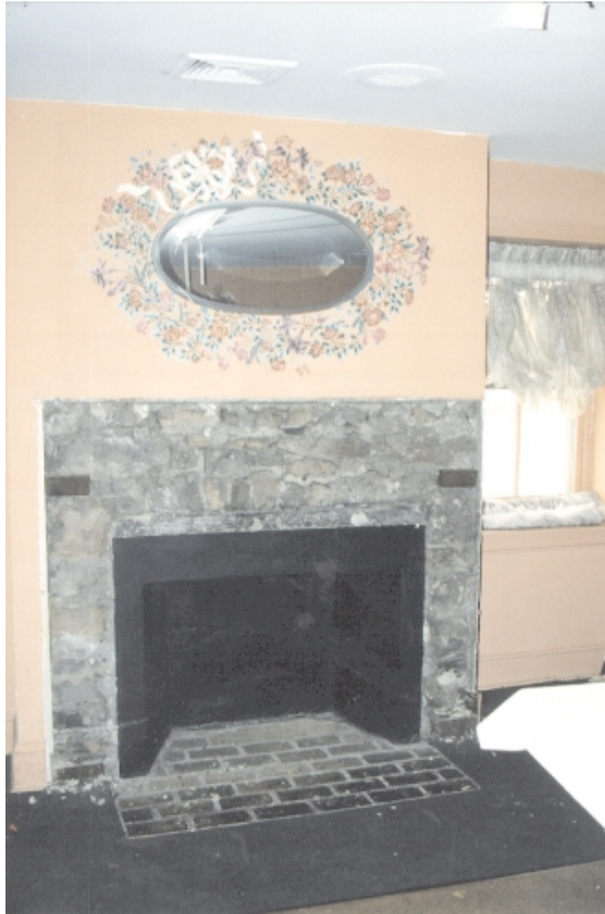
North wall second floor fireplace (Doug Crompton 12/6/97)
