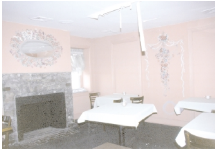
Second floor general view to northeast corner (note fireplace and window openings) (KAA:97-15/17) 12/6/97
