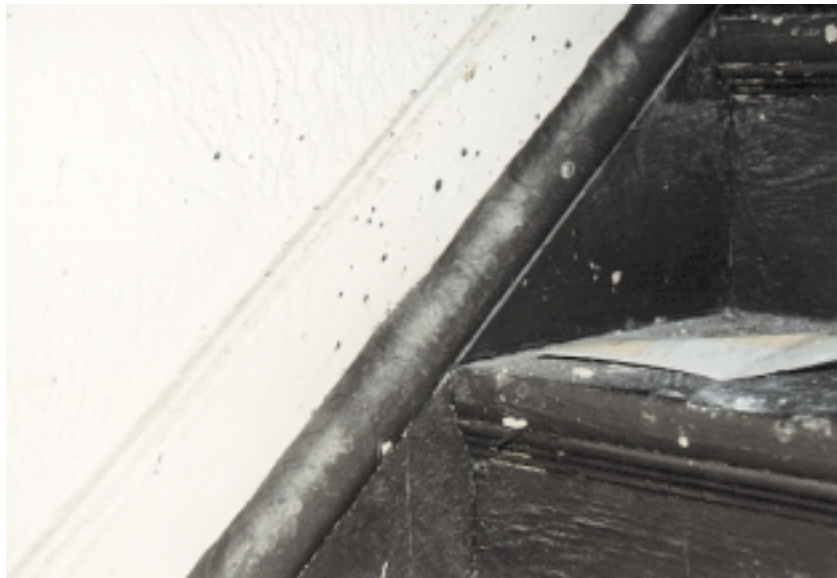
Stairwell to attic, stair tread and baseboard detail (Doug Crompton 12/6/97)
