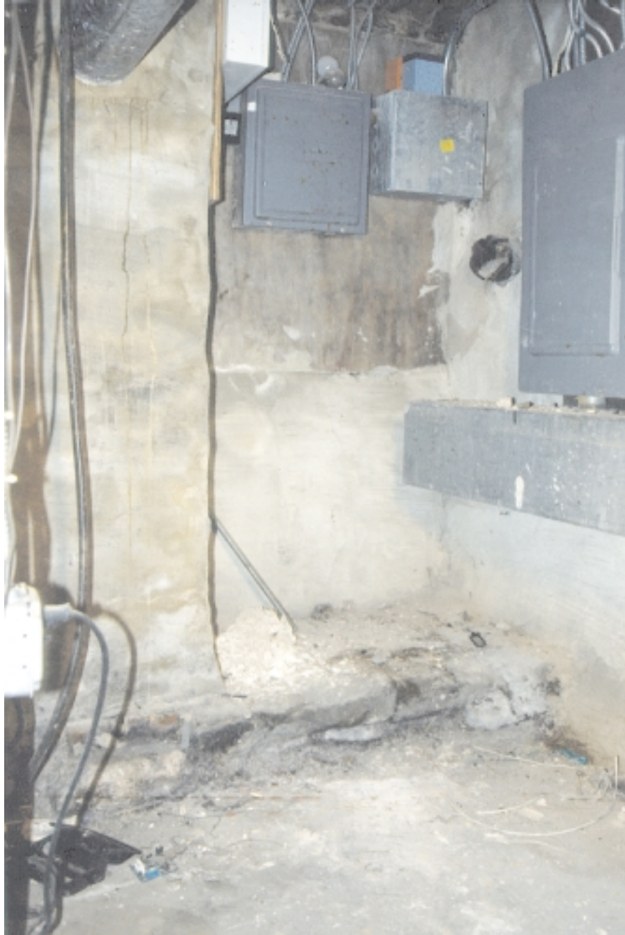
Basement alcove, view back to northwest corner of regular basement, closed window? (Doug Crompton 12/6/97)
