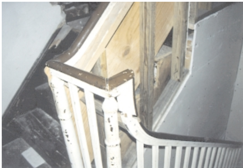
Stairwell to attic, landing detail balusters, newels and railing (Doug Crompton 12/6/97)
