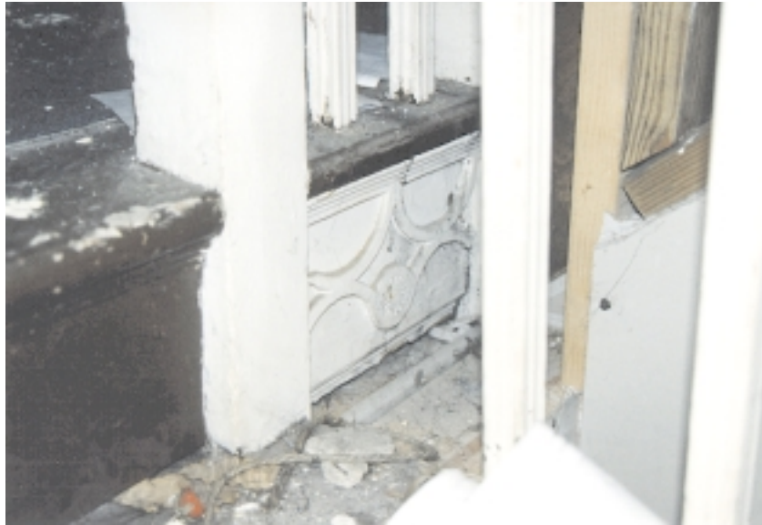
Stairwell to attic. Fretwork detail at landing (Doug Crompton 12/6/97)
