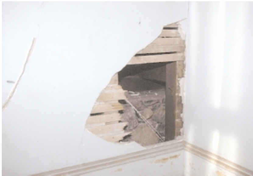
West attic wall, top of original stone wall behind plaster (KAA:97-15/10) 12/6/97
